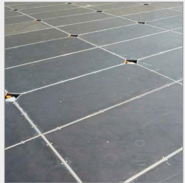
Destil Deck Infill Caps are a very easy tools in order to close the gaps between the perimetral (wich means the perimeter of props span module) Alu Panels joining in correspondence of Drop Heads.
